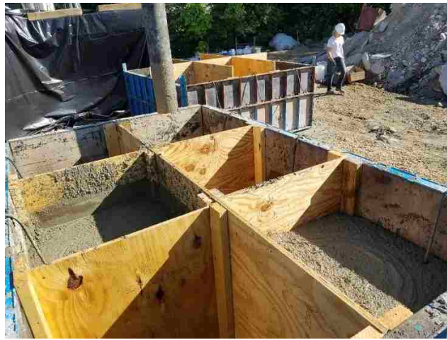
Figure 4-8 Formwork used to discharge pumped concrete.
